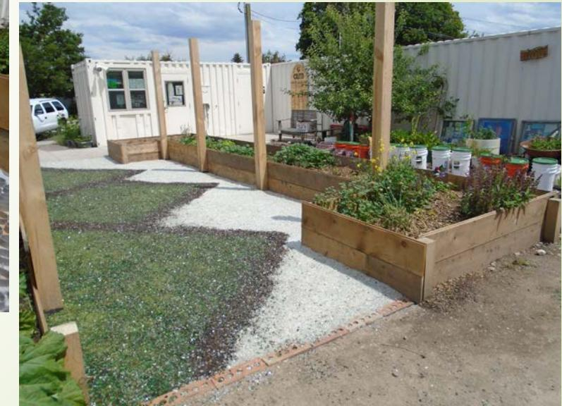
MUD purchased and installed a Gravelpave2 and recycled glass pathway.
