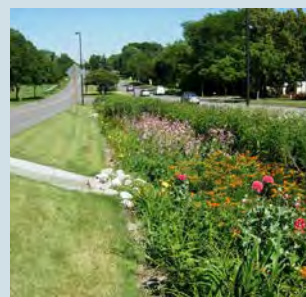
Bioretention Swale
