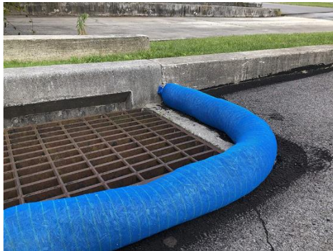
Filter sock for catching sediment. Photo credit: newpig.com
