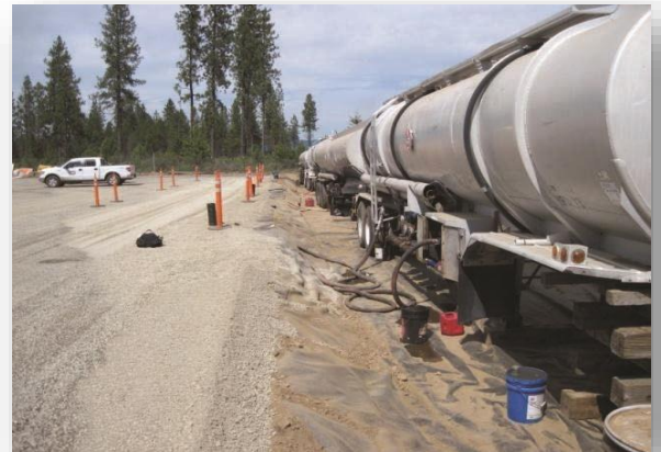
Temporary fueling site with liners under both storage and offload/onload lane (Note black inspection ports along lane). Photo credit: Panhandle Health District.
