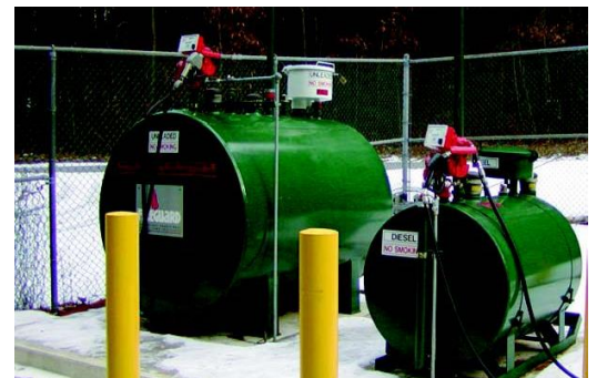
These ASTs are mounted on level impermeable ground with barriers to prevent vehicle collisions. Photo credit: Purdue Extension.
