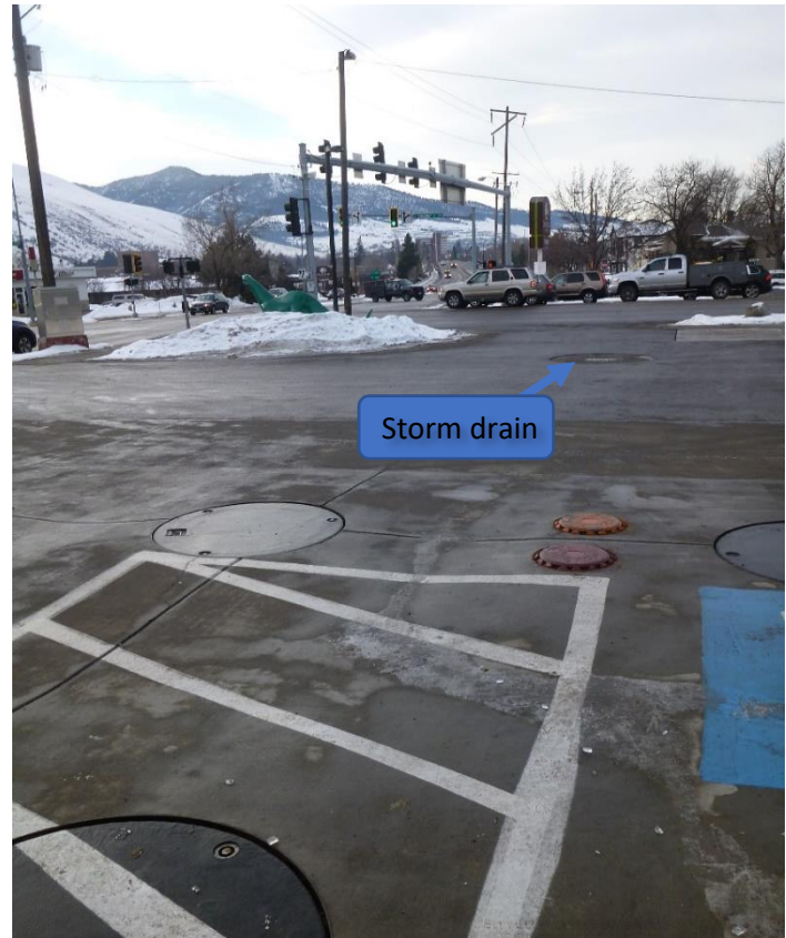
Dry well located directly downgradient from tank fueling area. Another storm drain along the road curb is also downgradient and leads to an outfall on Rattlesnake Cr.
