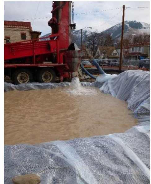
Sediment basin during well development. The rate of filling of this basin exceeded sedimentation. Filtration was necessary prior to discharge to the stormwater system.
