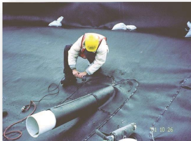
Technician seaming a 'boot' in a liner perforation. Photo credit: Panhandle Health District
