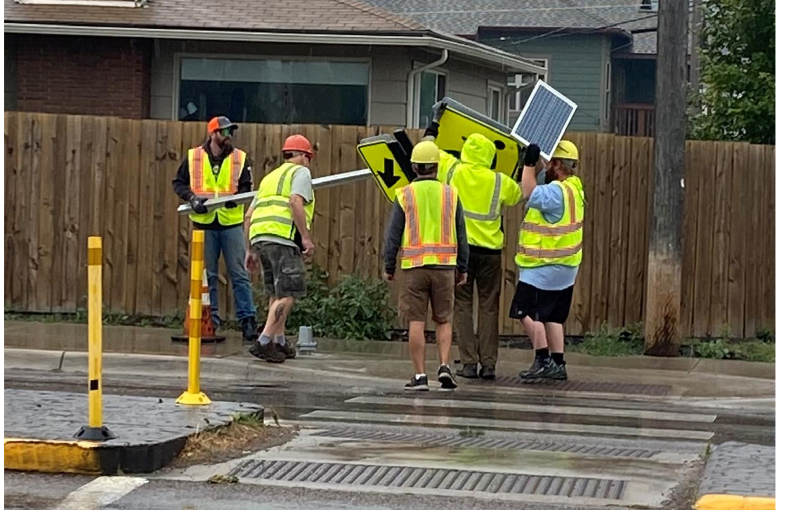
Traffic Services crew installing a Rectangular Rapid Flashing Beacon (RRFB)
