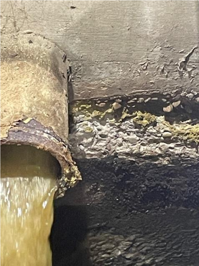
Corroding concrete at headworks
