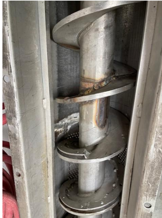
Washer/compactor screw and perforated pans require repairs
