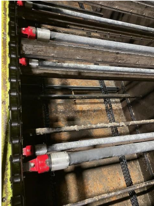
DAF chains in service since 1975 need to be replaced
