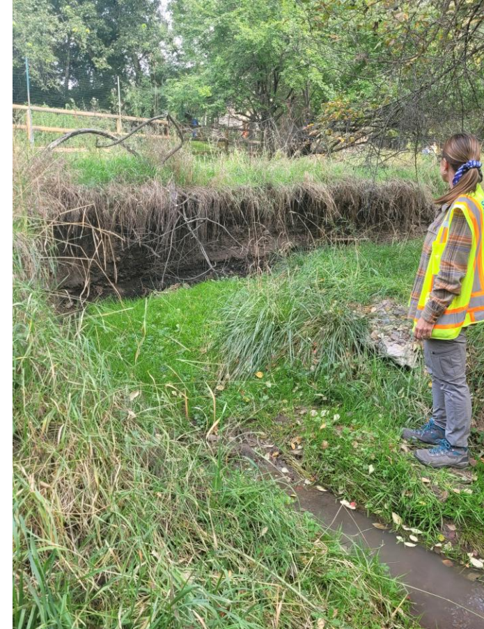
Headcutting and erosion in High Park drainage
